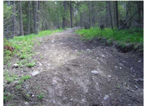
Unauthorized road for motorized use in KM sub area
